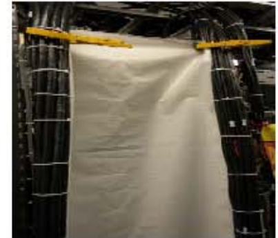
Use of Flame Retardant Plastic Sheetting as a Barrier
