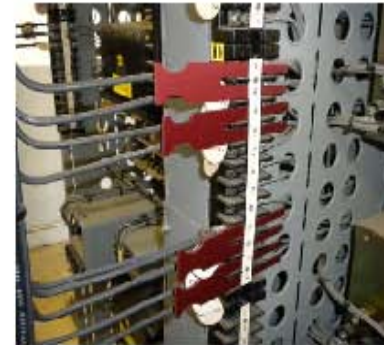
Use of Terminal Point Barriers
